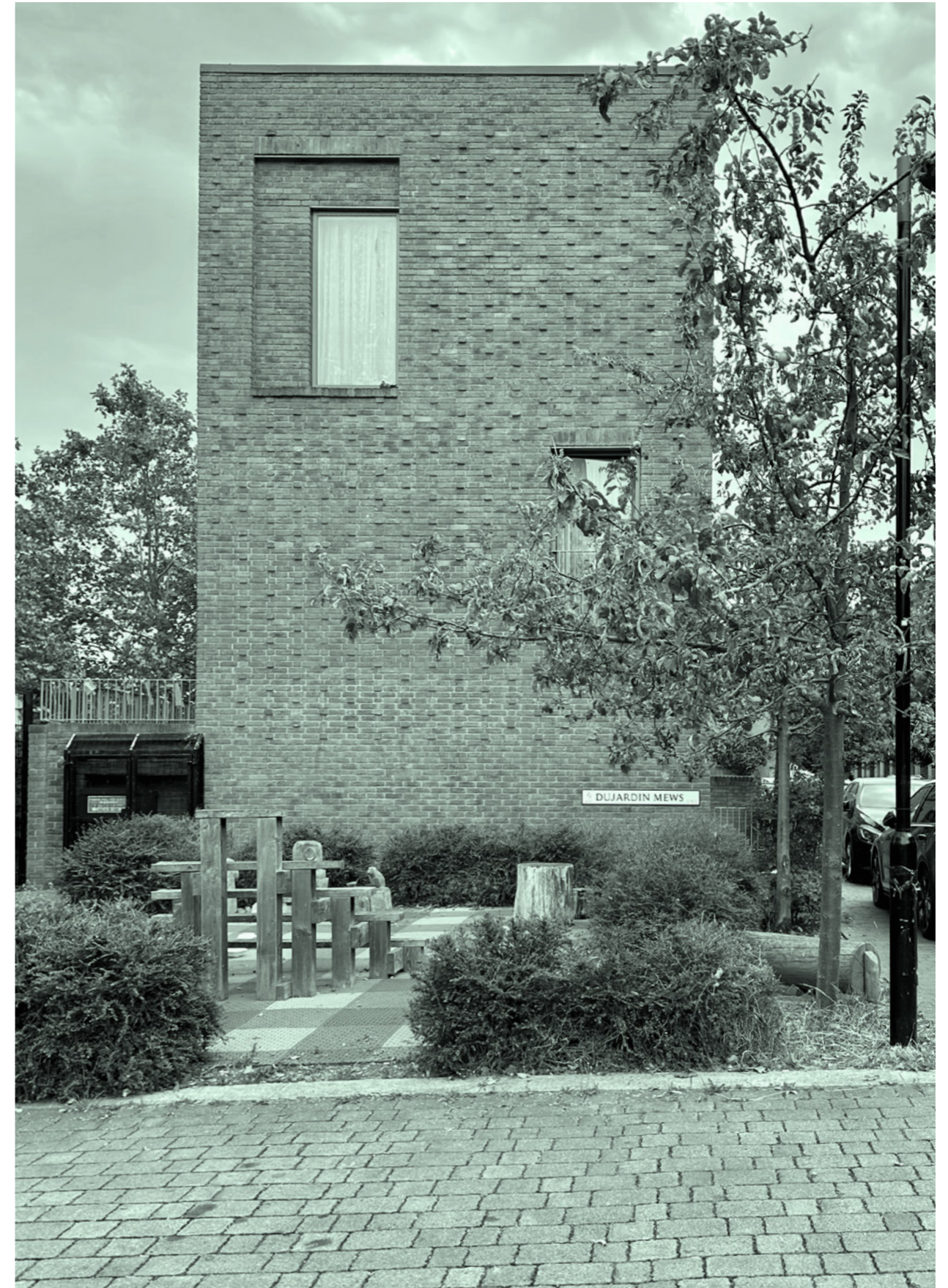
Dujardin Mews, Enfield, Karakusevic Carson with Maccreanor Lavington Architects and East Architecture Landscape Urban Design (2017) Map Location →
