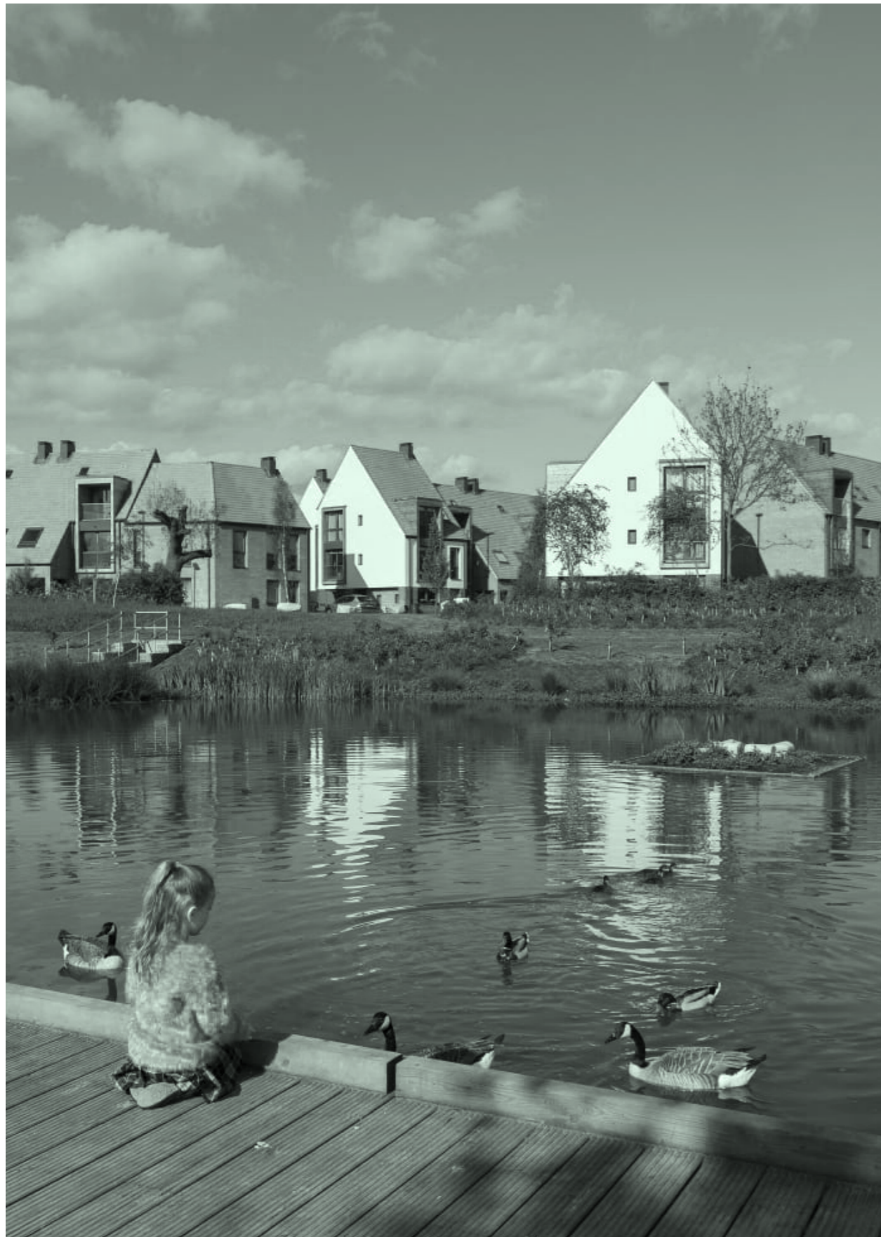
Derwenthorpe, York, Studio Partington with FIRA Landscape Architects and PRP Architects (2019) Map Location →
